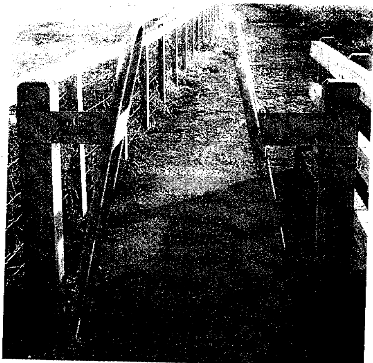
Galvanized steel access control barrier supplied by FEARN (Truck Bodies) Ltd of Rotherham to be installed at bridge entry points. Barriers are 1500mm high, and fixed to 150x150 H/W posts 1200mm high. Gap at base is 1000mm, narrowing to 350mm at top. Designed to permit access by cyclists and wheelchair users but prevent entry by motorcycles and horses
